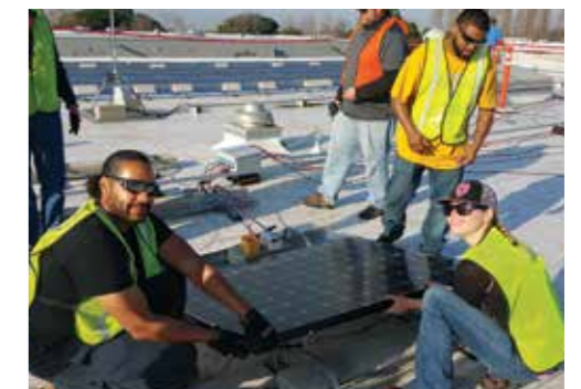
Teamwork to take this roof solar
